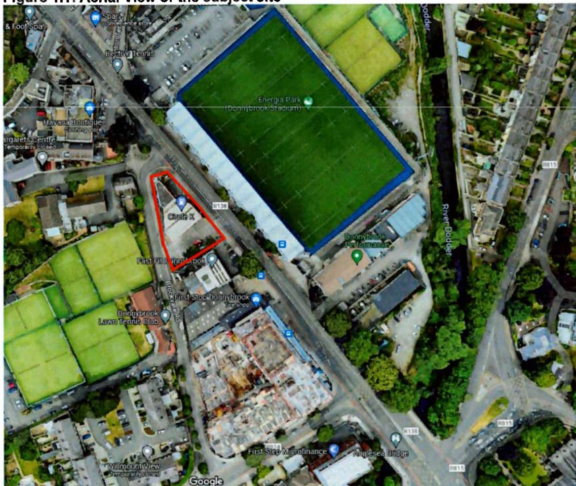
Figure 1.1: Aerial View of the subject site
